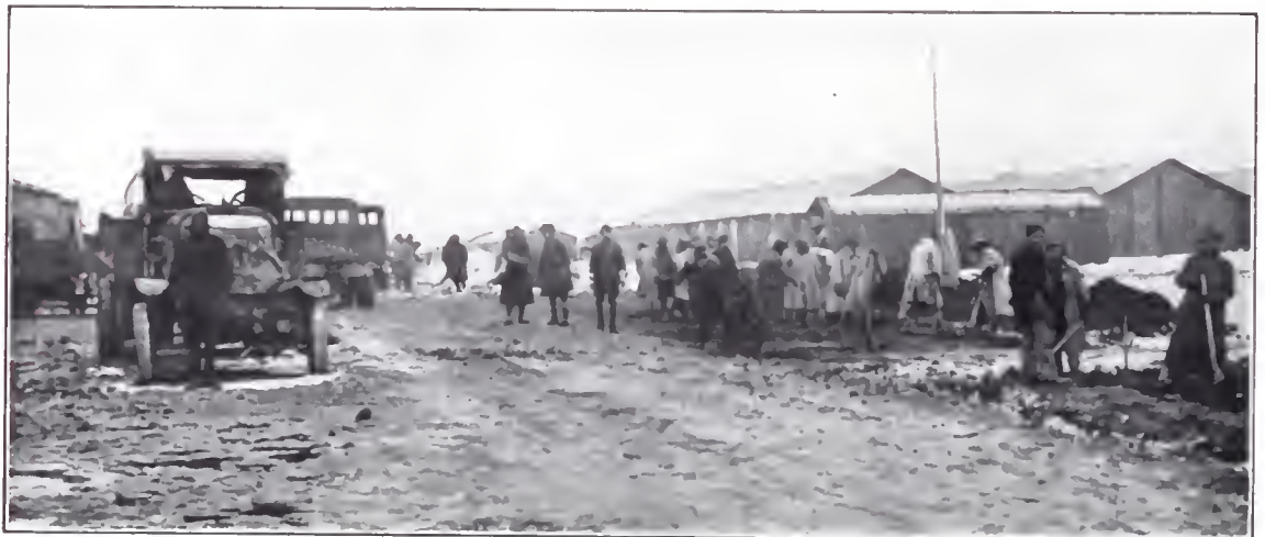
Road Building, Mesves Hospital Center.
