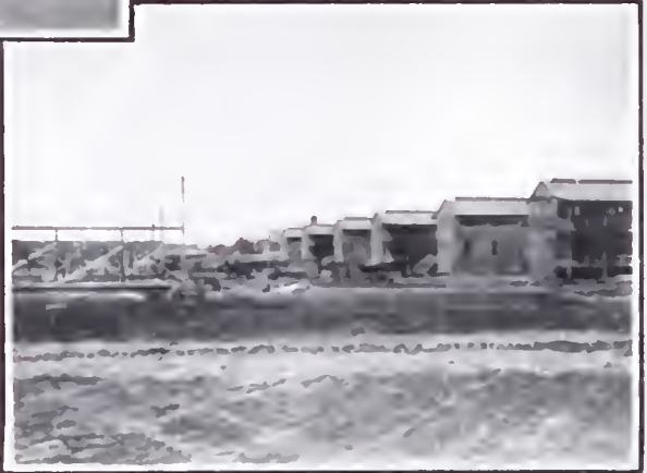
New Hospital Buildings, Temporary Barracks for Enlisted Men of Base Hospital No. 44. Camp Dix
